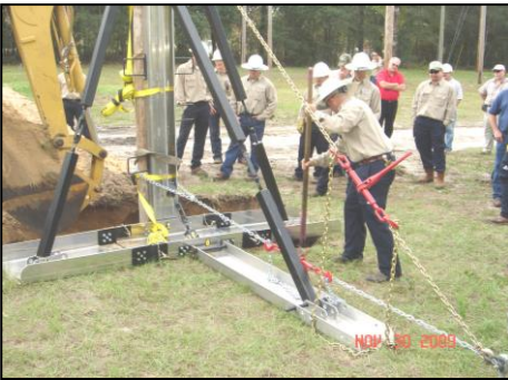
Removing sand from underneath base
