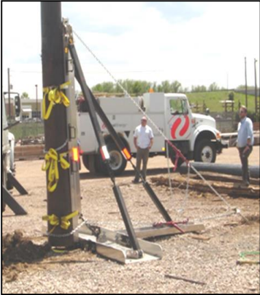
Pole attached to free standing Ver-T-Pol
