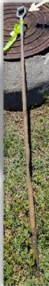
Electric utility's helix anchors
